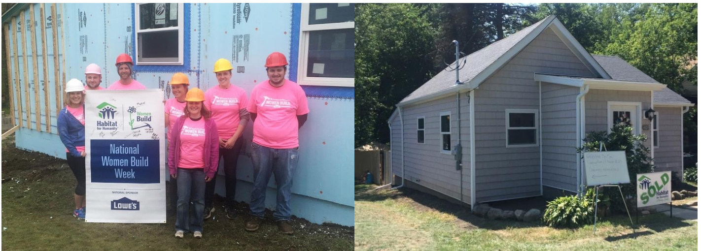
Figure 24: This 1890 home near Lake Erie was retrofitted by Habitat for Humanity volunteers to be all-electric and comfortable in all seasons. 66
