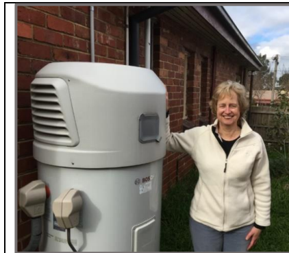
Figure 40: Jane Fisher decided to install an energy saving heat pump water heater at her investment property in Melbourne. 88
