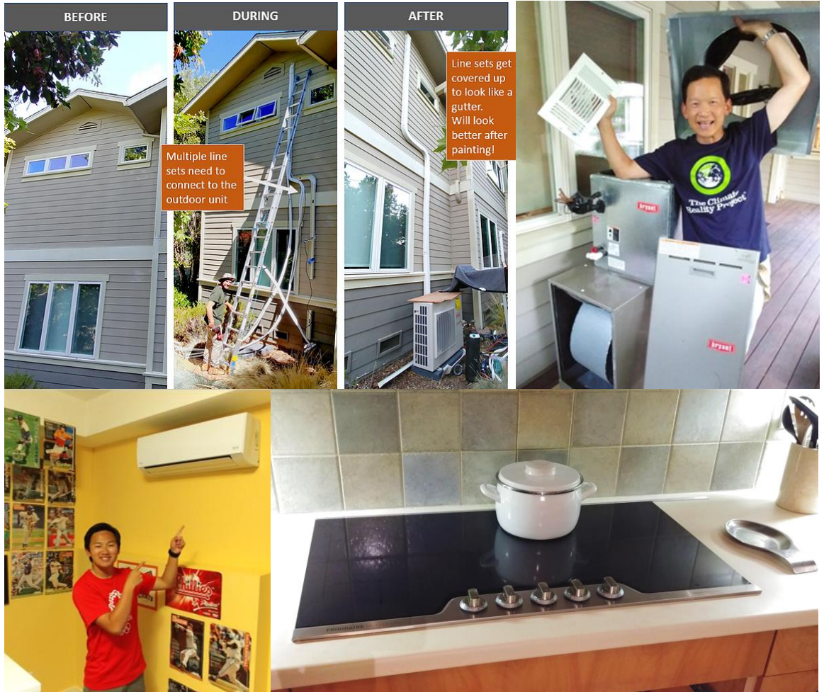
Figure 28: Out with gas and in with electric mini-splits and induction cooking! 71
