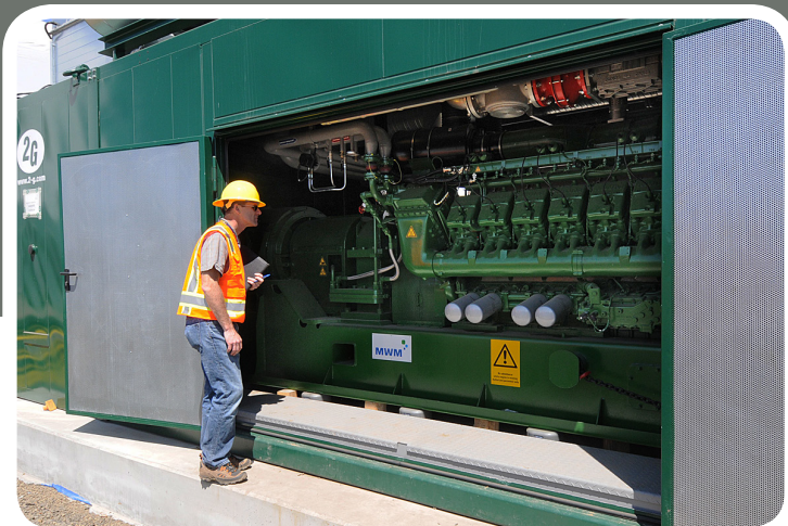
A look at the engine inside the co-generation unit and some of its 16 cylinders. The engine turns a generator to create electricity.
